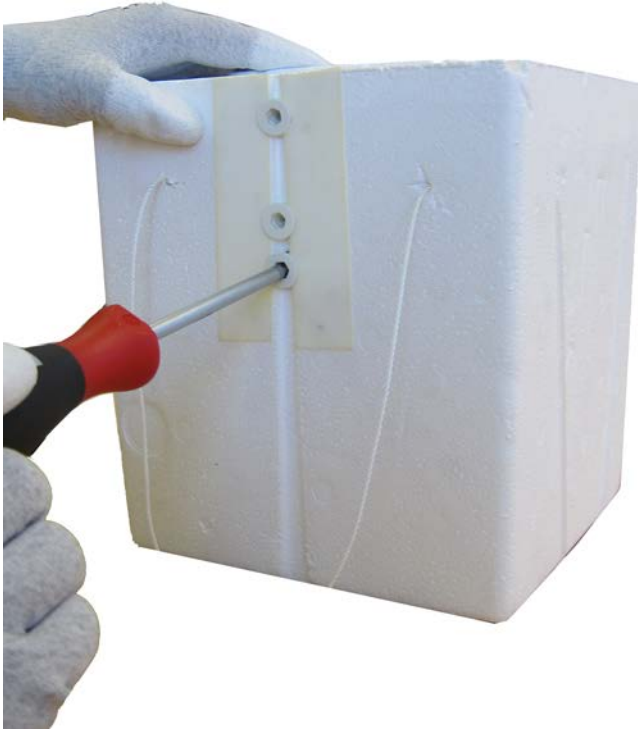
Figure 18 Inserting the Dowels
